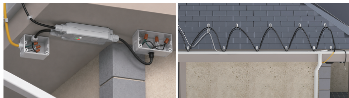
Roof / gutter / eave installation area
